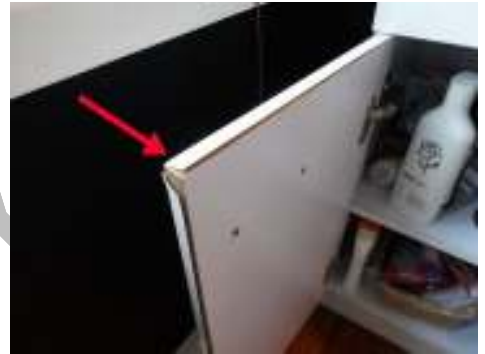
Door cover delaminating.
