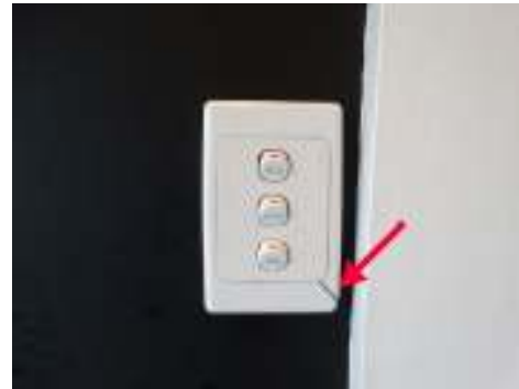
Cracked switch.
